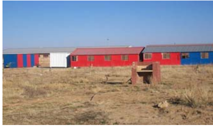
Drop-in centre at Nellmapius is housed in two former shipping containers.
