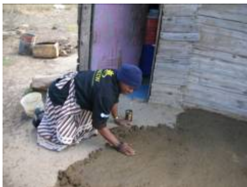
A child care worker 'cementing' a floor with cow dung at a home of a family.
