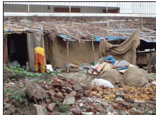
Roofs covered with branches
